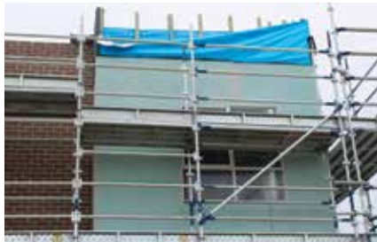
FIGURE 3.22 Jointing & Coating System
