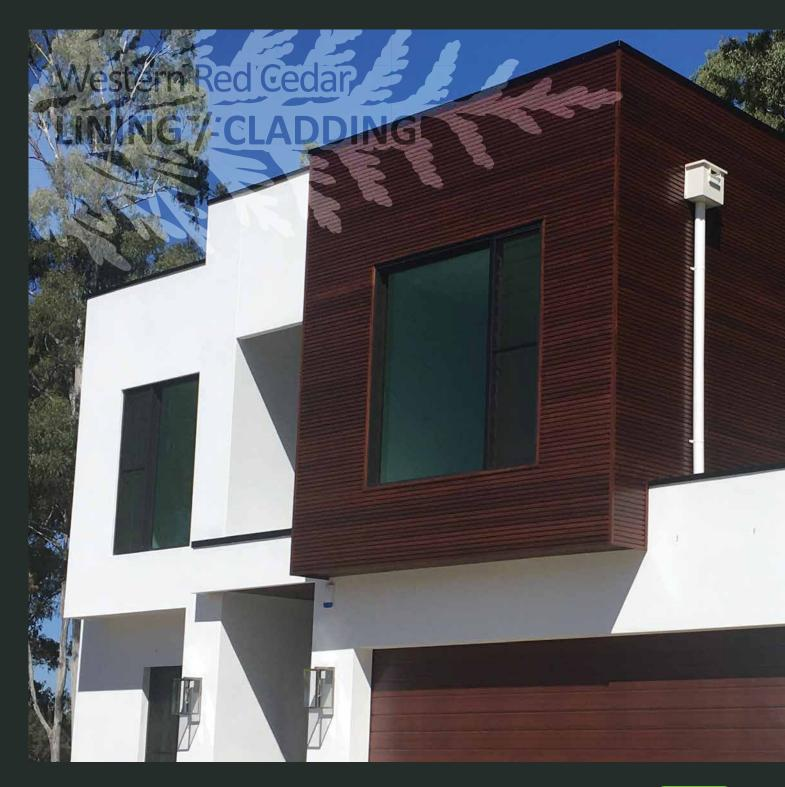
Horizon<sup>™</sup> provides a continuous, bold, linear appearance with strong shadow lines – making it ideal for interior and exterior feature walls. The castellations on Horizon's surface create the effect of dressed battens, with the convenience of secret nail tongue and groove profiling.
